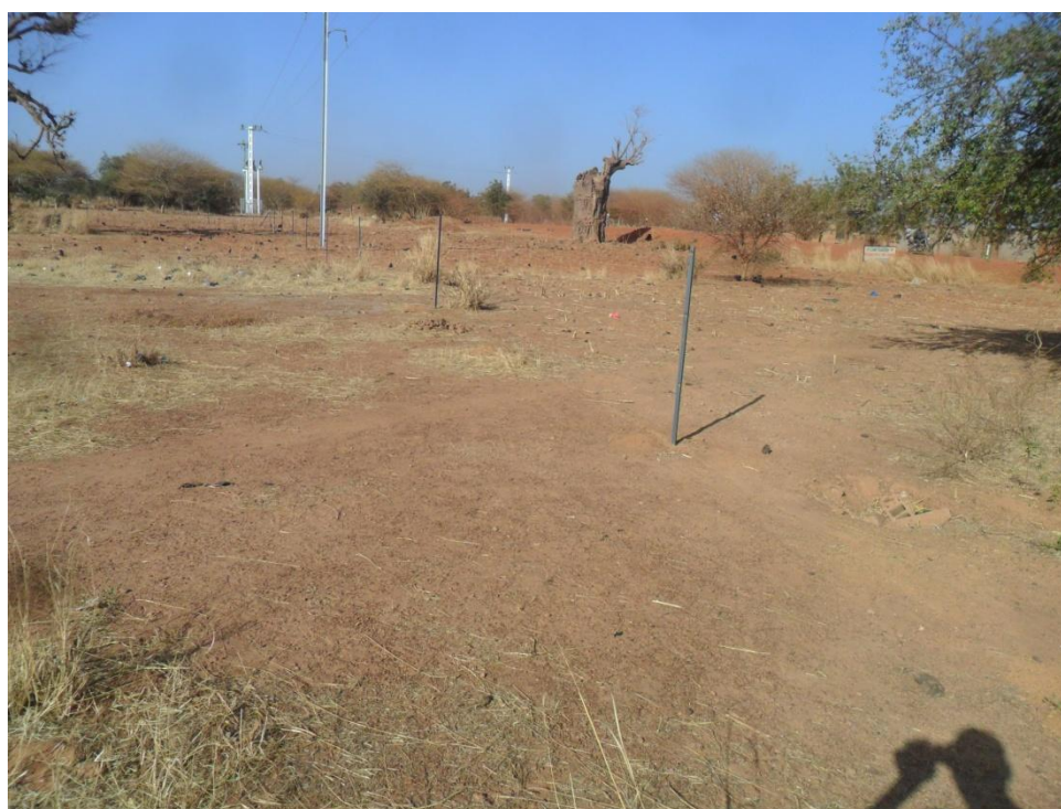
Installation des poteaux
